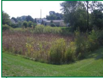
A portion of the Caddell Drain Storage Facility in Farmington Hills.
