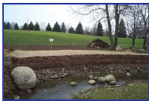
Plymouth Township completed streambank stabilization along various sections of Tonquish Creek.
