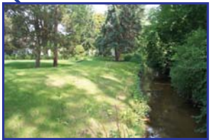
The City of Novi received Rouge Project funding to conduct a streambank stabilization project using bioengineering upstream of the Northville Mill Pond.
