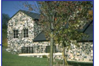
Linden Park in Birmingham is the site of one of three combined sewer overflow control basins in Oakland County.
