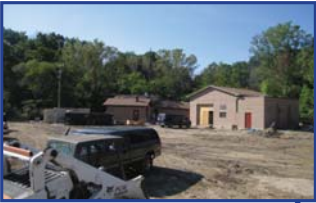
Construction of the Walnut Lake Pump Station in West Bloomfield Township .
