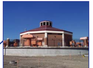
The CSO Basin in the City of River Rouge became operational in August 2002. This basin was designed to capture the 10-year, 1-hour storm and has a capacity of 5.2 million gallons. All ten of the CSO retention/treatment basins planned for Phase 1 of the Rouge Watershed CSO control program are now in operation.
